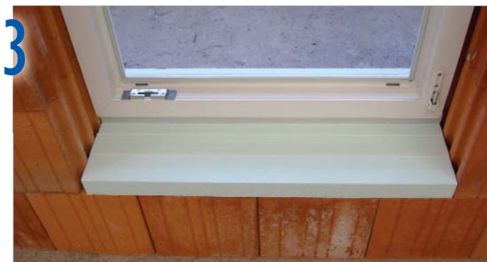
Set the window frame with attached L profile and caulk in place
