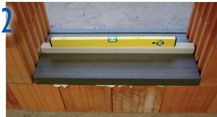
Glue the Thermo component in place and align it
